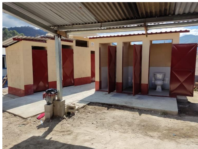
A newly completed school sanitation block with separate girls changing room for MHM (left rear of photo)
