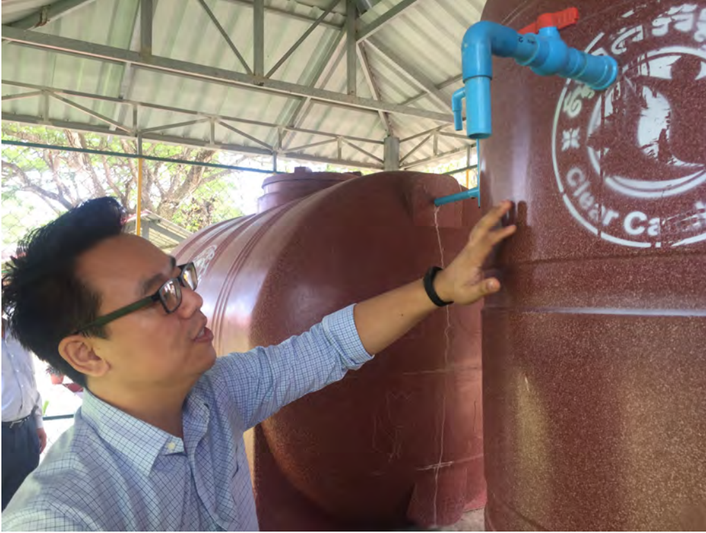
charity: water staff Steve Che describing the filtration process. The system is gravity fed and the water is piped into the first tank and then starts the process of filtration. The BioSand filter removes 99% of bacteria!
