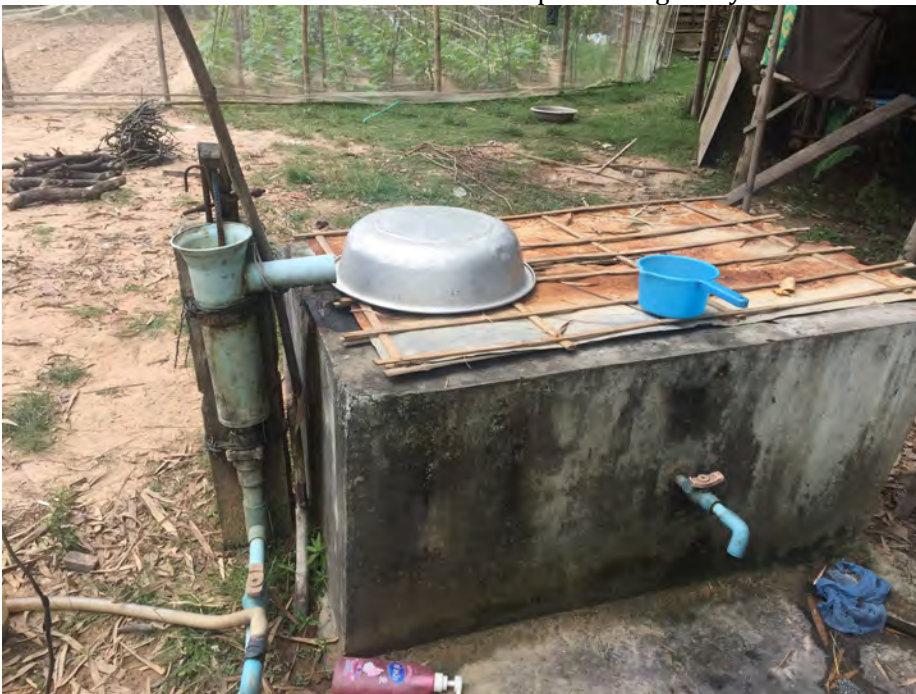
Well/rain catchment system which is the source of the family's water. A few houses now share the BioSand filter for their clean water needs.
