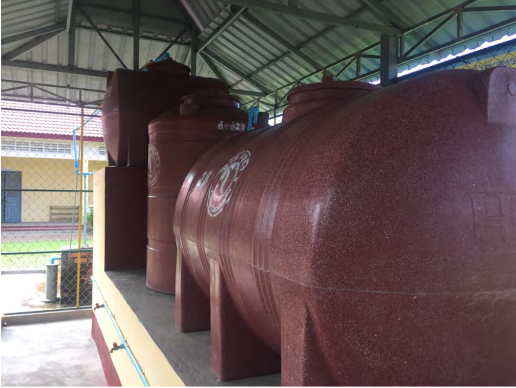
Large school Biosand Filter. Capable of delivering clean water to over 1000 people
