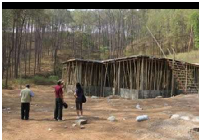
Dhankuta Clinic 1 st floor construction May 2012
