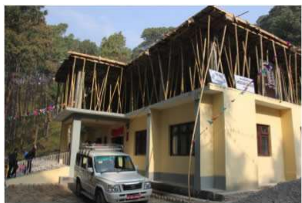
December 14, 2013 Inauguration Day_2nd floor started
