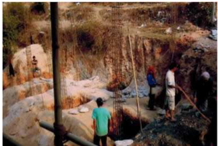
Pouring the foundation July 2012
