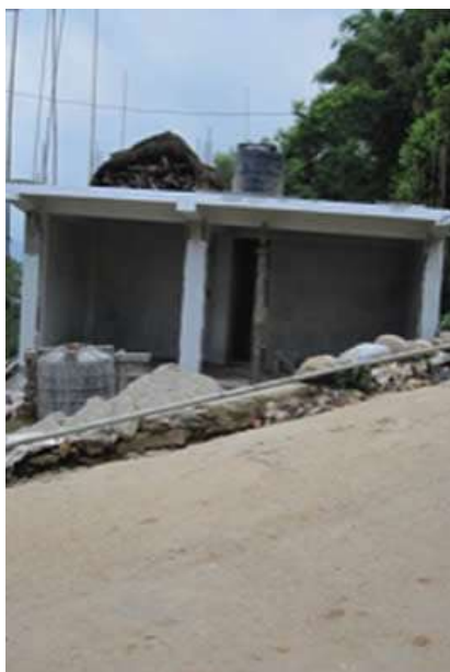
Clinic construction starts September 2013
