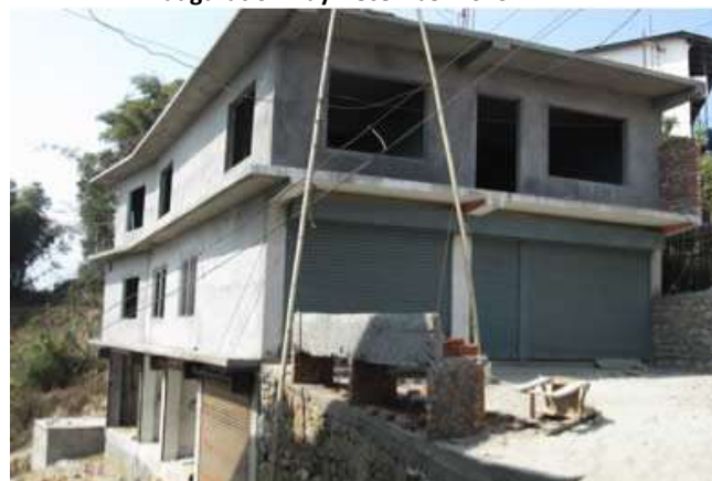
Third Floor construction March 2014
