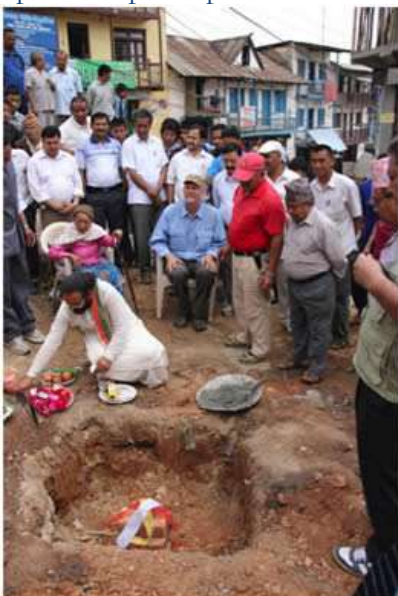
May 2012 Khandbari Laying the corner stone
